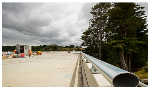
Texas handrails installed on Arawhiti ki Ōkahu.
