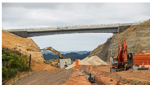
Longitudinal drainage at Tapuwae o Kahumatamomoe.
