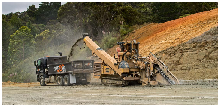
Trenching machine in action.
