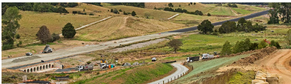
Completed farm access and batter stabilisation in the north of the project.
