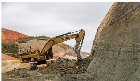
Trimming of rock batters.
