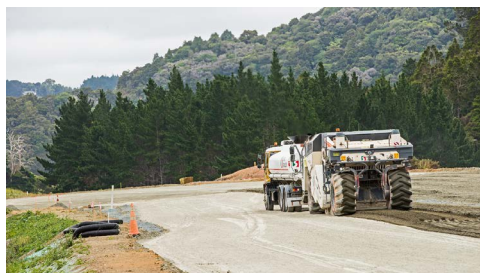
Stabilising the subgrade improvement layer.
