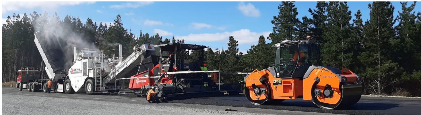
This photo shows the paving machine laying asphalt on in the south of the project during asphalt trials.
