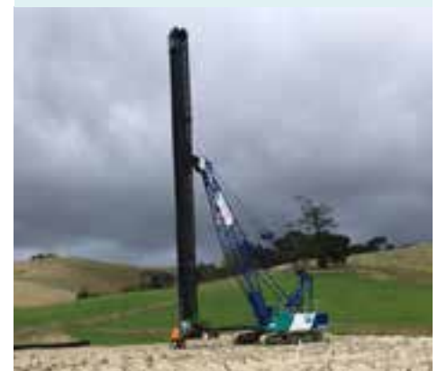
Preparation begins for a trial embankment off Wyllie Rd.
