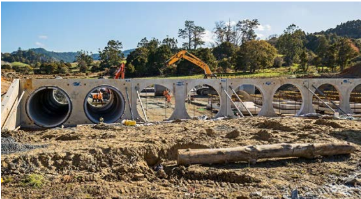
11 Barrel Culvert – North. This will be the biggest culvert to date in New Zealand consisting of 187 concrete pipes weighing 10 tonnes each. Each barrel will be 42m long and 2400mm in diameter
