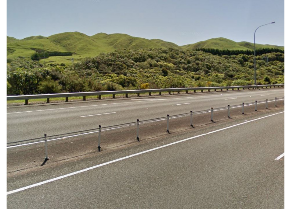
Motorway through rural land 1
