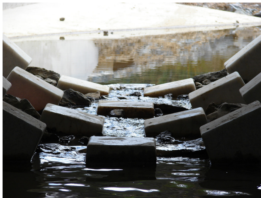
Baffles within a culvert 1
