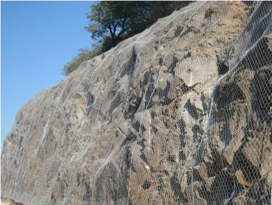
Rock mesh and bolts to be used along the tops of cuts
