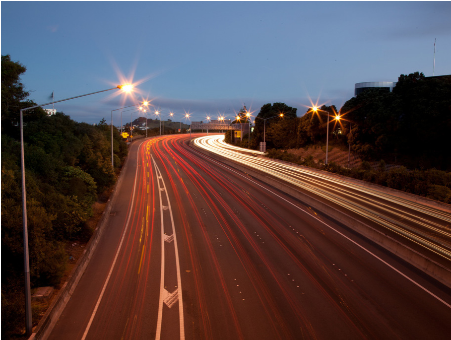
Example of mitred street lights (Southern Motorway at Grafton Road) 2
