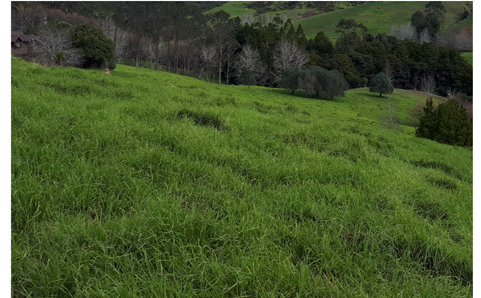
Example of a hydroseeded fill slope
