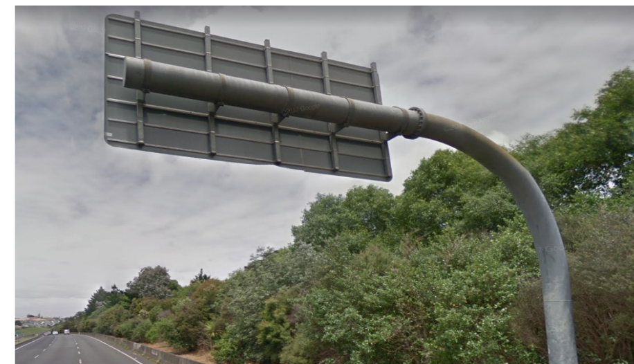
Example of a cantilevered sign gantry 1
