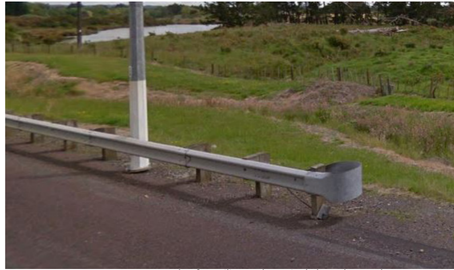
Example of a trailing end terminal along the Southern Motorway 1
