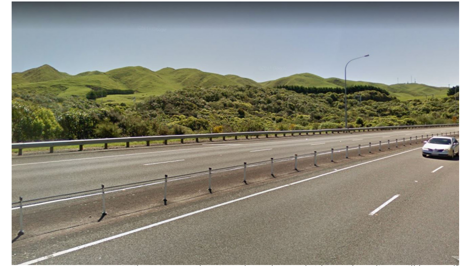
Similar wire rope barriers along the road sides and medians will be used 2
