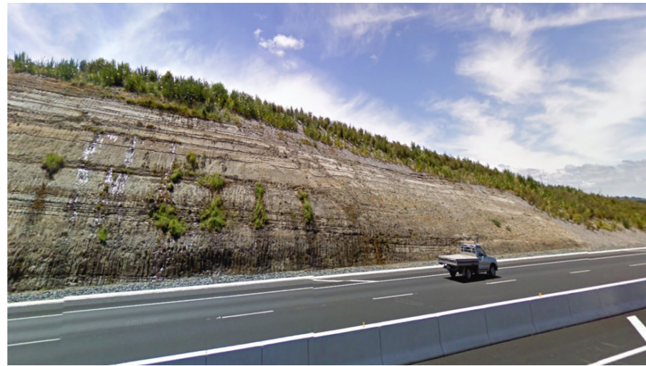
Cut slopes on the Northern Gateway Toll Road which are similar in nature to what will occur 1
