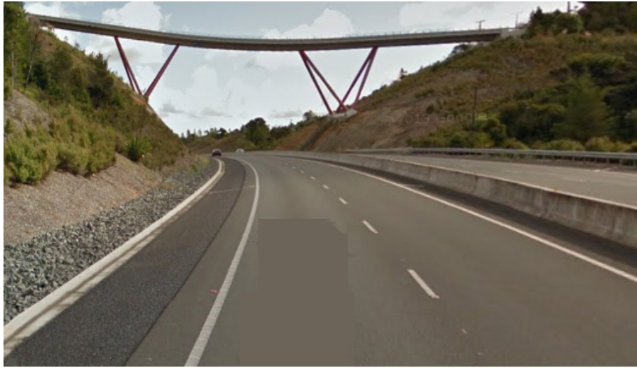
Kerb and channel on the Northern Gateway Toll Road, similar to that used on the Project 1
