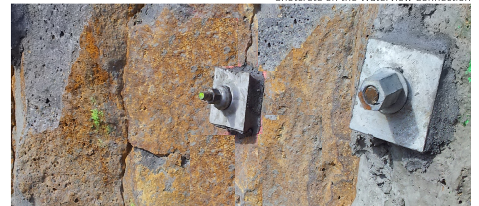
Rockbolts used on the Waterview Connection
