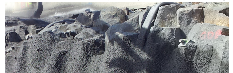
Shotcrete on the Waterview Connection
