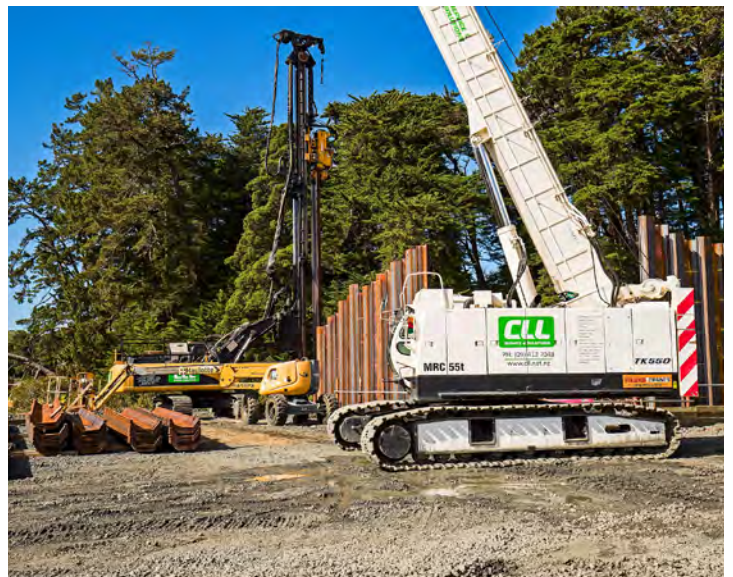
Sheet piles being installed at Te Arawhiti ki Ōkahu
