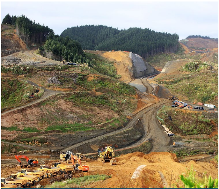
View from the purpose-built viewing platform, overlooking some of the project's most significant cuts and fills. Here people could start to see the new motorway taking shape and gain a first-hand appreciation of the scale of the project.
