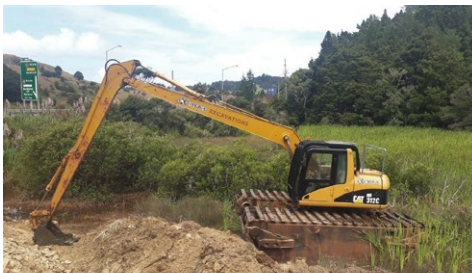
Amphibious excavator at work near the Pūhoi River
