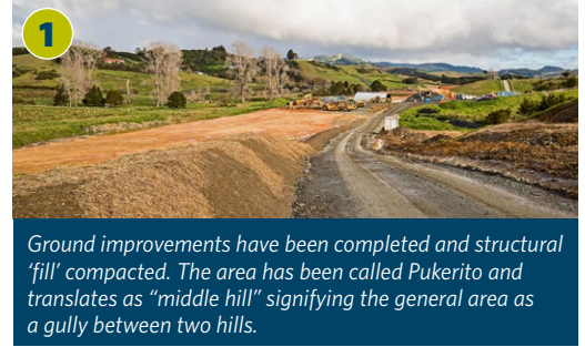
1 Ground improvements have been completed and structural 'fill' compacted. The area has been called Pukerito and translates as "middle hill" signifying the general area as a gully between two hills.
